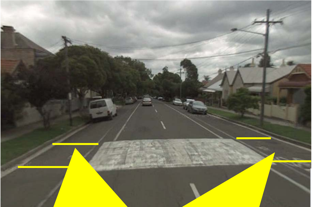
Cyclist and pedestrian route improvements...extension of speed humps in Renwick Street, Drummoyne
